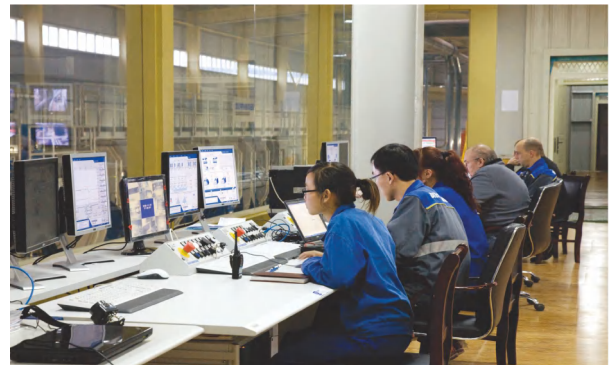
Control centre (produced according to European EN300 standards)
