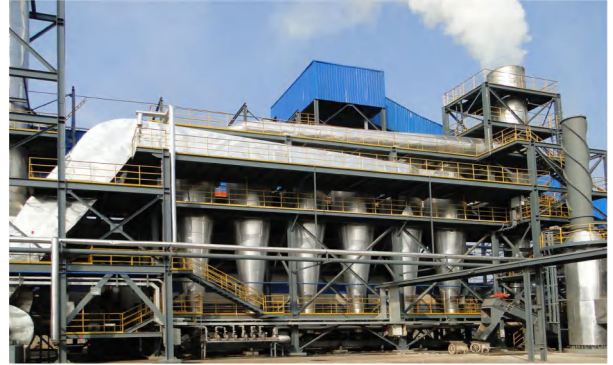
GTS Thermal Power Plant
